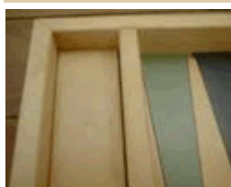
Corner section showing glued and screwed checker housing
